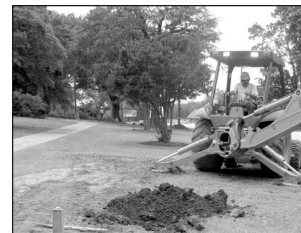
Construction workers prepare the grounds for the new signage on Hwy 76
