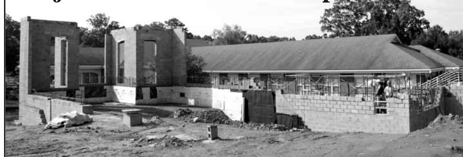
Walls of the new pool building begin defining the space
